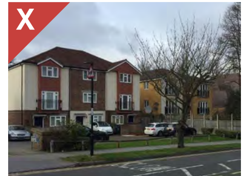
Figure 2.17d: A development which appears wide and squat as a result of poorly considered proportions and fenestration
