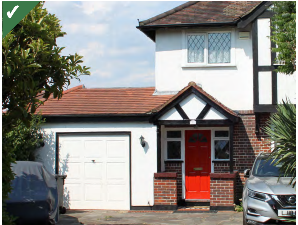
Figure 4.14a: Example of a good side extension wrapping around to incorporate a well-designed porch, successfully integrating with the existing dwelling.
