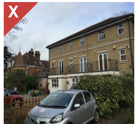
Figure 2.24b: Windows are too small and their positioning fails to break up mass of façade.
