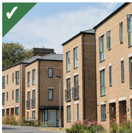
Figure 2.27b: Example of where placement of servicing items has been considered early in the design development, ensuring elevations are kept free of clutter.
