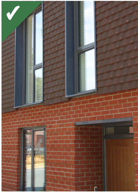
Figure 4.25a: A wall with different depths of window and door reveals. Deeper reveals add emphasis and solidity to the appearance of a house.
