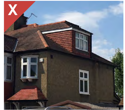
Figure 4.21e: Example of where a side roof extension to a house has not been setback from the original roof. In this situation it has compromised the symmetrical form of the original semi-detached houses and therefore negatively impacts the appearance of street.
