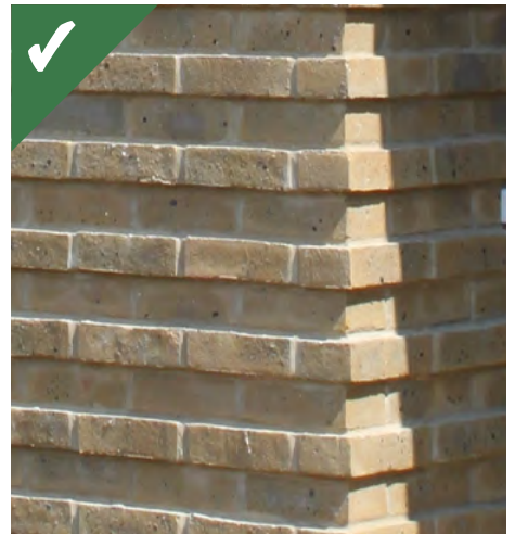
Figure 4.27e: Stepped courses of brickwork.
