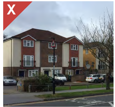
Figure 2.24a: Proportions and positioning of windows add to horizontal emphasis of the façade and contribute to a weak pastiche.
