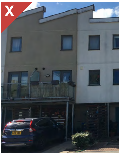
Figure 2.26a: External balconies with supports that are not integrated into design of the proposal. The use of glass balustrades have resulted in occupiers retrofitting screening devices to provide privacy exacerbates the poor appearance.
