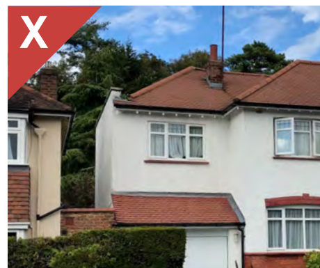
Figure 4.24c: The combination of a pitched roof with a parapet results in an unattractive appearance.
