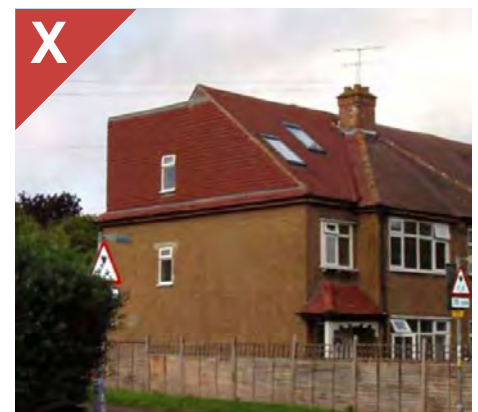
Figure 4.21g: Example of where a highly visible roof extension dominates the original building and negatively impacts the appearance of the street. This could have been avoided had the rear box extension been set in from the gable end of the roof to allow the gable and the rear extension to read as two separate elements.
