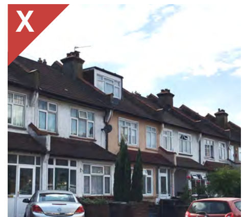
Figure 4.21f: Example of an inappropriate addition of a front dormer to a mid-terrace house. This addition lacks design merit and breaks the uniformity of the roofs that contributes to the positive characteristics of the street.
