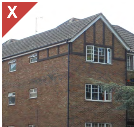
Figure 2.23k: Half-timbering has been wrapped around the side of the building but stops at the first window, highlighting that it is non-structural and is an applied detail. It should have either been continued along the length of the building or kept within the gable so it did not break the eaves line.
