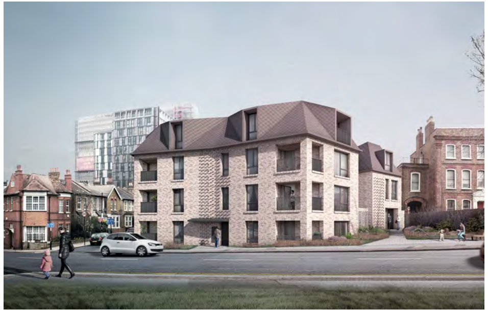
Figure 2.8b: Coombe Road - an example of a Contemporary Reinterpretation approach designed by Common Ground Architects. The massing and materials of the proposal refer to the surrounding buildings, but distinguishes itself through the folded form of the roof and contemporary detailing. The proposal delivers several new homes across two buildings.
