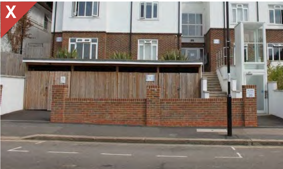
Figure 2.31c: Refuse stores in highly visible locations that are not integrated into the landscape design or any other aspect of the design.
