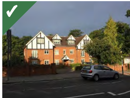
Figure 2.17c: A wide development which has successfully dealt with its width through proportions and fenestration
