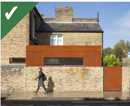
Figure 4.26c: An example of the successful introduction of contemporary materials in this metal clad side extension by HUT Architecture.
