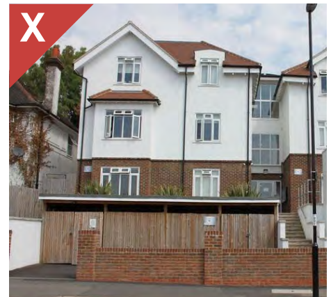
Figure 2.29b: Failure to screen hardstanding and bin stores with a landscaped boundary treatment.
