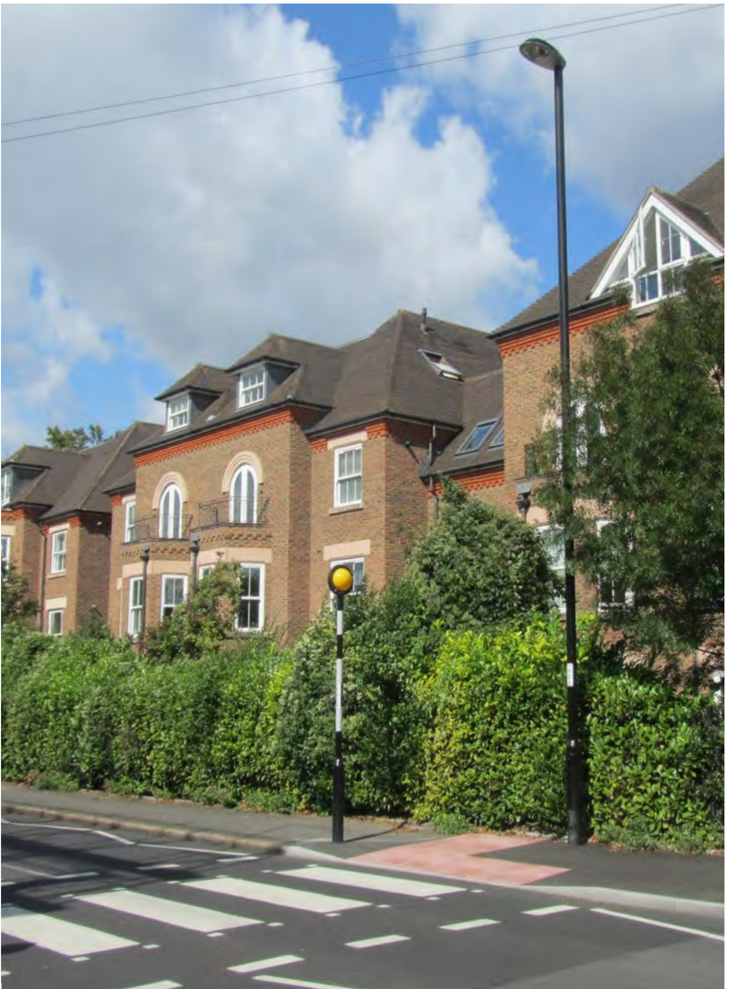
Figure 2.13d: A development of flats that faces onto the Croham Road is 4 storeys tall, with 1 floor contained with the roof. The development is formed of blocks that refer to the scale of dwellings along the street with recessed linking elements. Refer to guidance 2.10 and 2.15.
