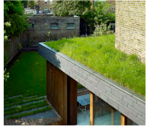
Figure 2.36a: Green roof designed by Hayhurst & Co.
