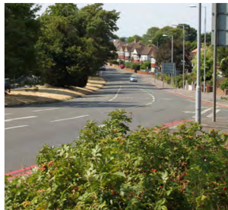
Figure 3.16b: A232 Dual Carriageway
