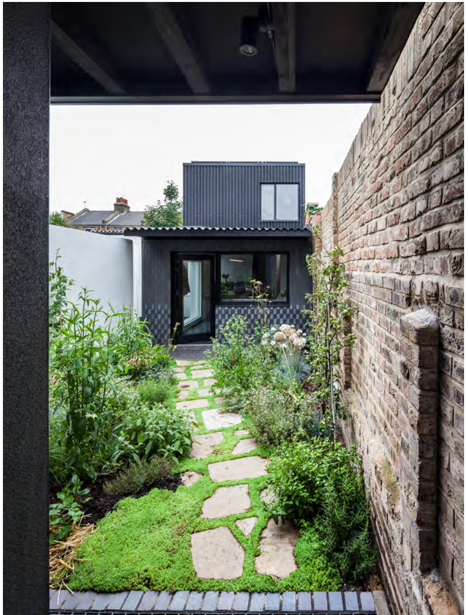
Figure 2.18a: A rear-garden house designed by Dallas–Pierce–Quintero that builds along the boundary wall. (Photo: David Butler)
