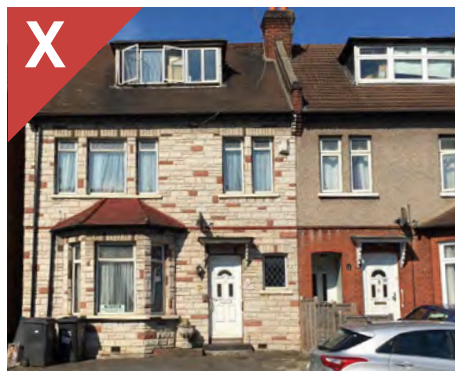
Figure 4.26d: An example of inappropriate cladding to a house that hinders the appearance of the street.
