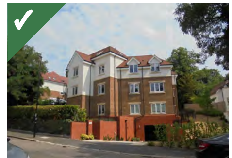
Figure 2.20e: Successful use of topography to integrate parking into a basement. Once matured, planting will reduce appearance of retaining wall.
