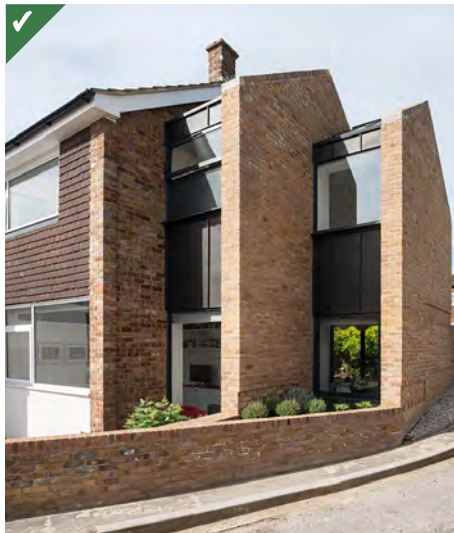
Figure 4.17c: Example of a subservient two-storey side extension designed by Selencky Parsons that introduces contemporary elements, such as the windows and their surrounds, to help distinguish the new from the existing. (Photo: Andy Matthews)
